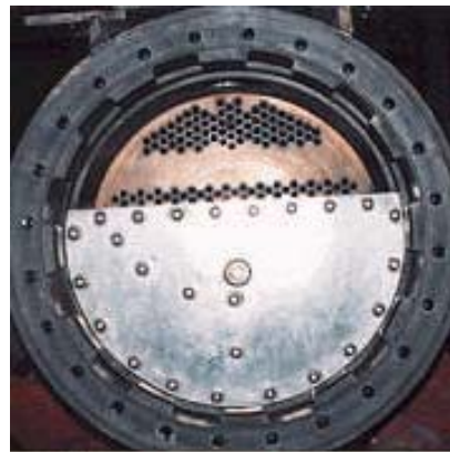
Figure 13 - Inspecting heat exchanger tube sheet and end plate for leaks
