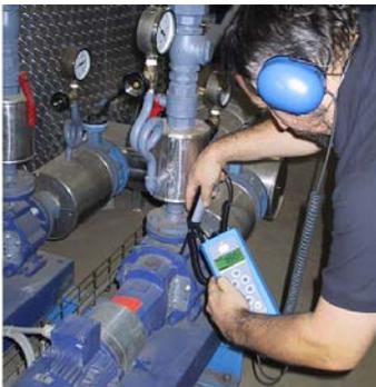
Figure 4 - Monitoring feed water pump
