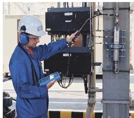
**Figure 3 - Conducting an air leak survey**
